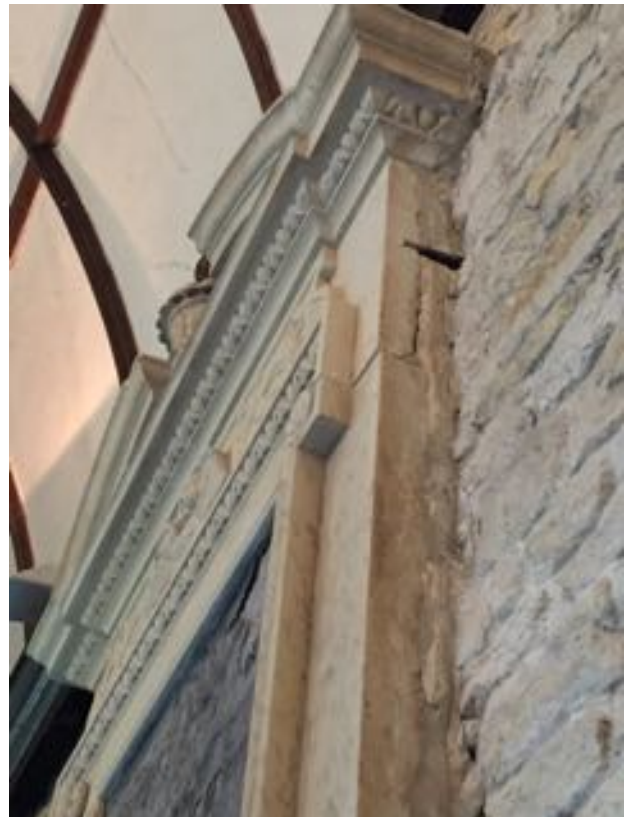
Figure 16 ~ Crack at high level along the side of the monument.
