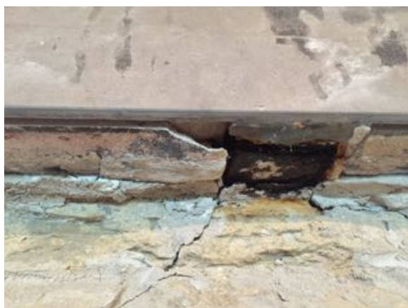
Figure 19 & 20 ~ Corroding ferrous armature causing monument to detach from wall
