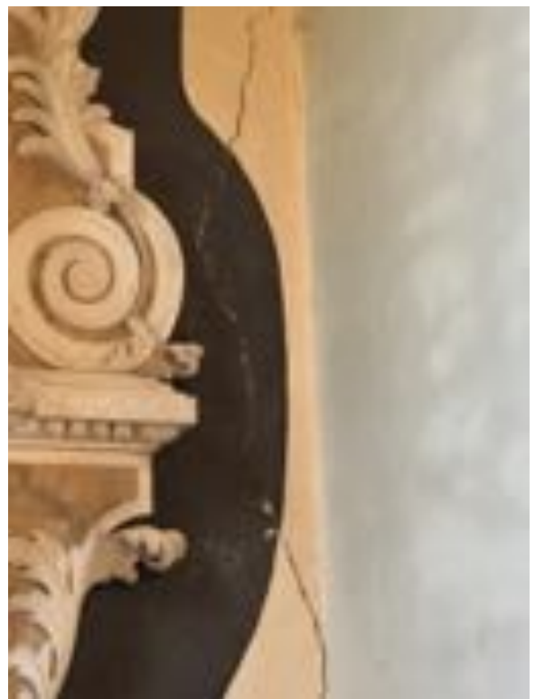
Figure 4, 5 & 6 ~ Details of cracks to the east and west of the monument, as well as extending across the ceiling.
