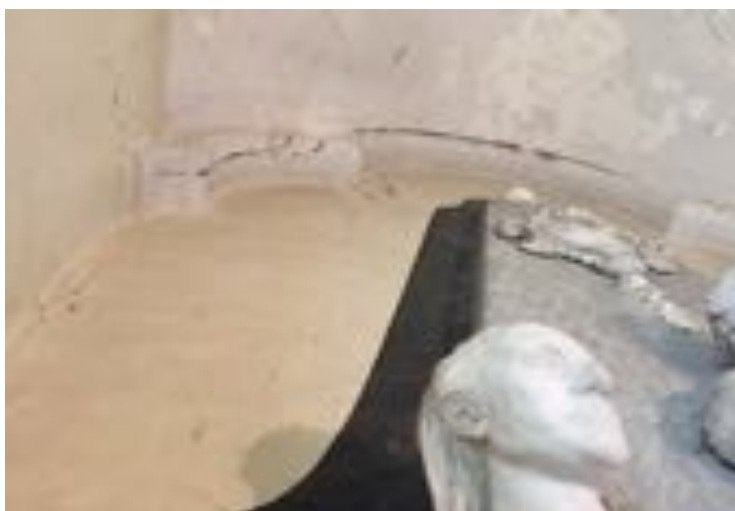
Figure 4, 5 & 6 ~ Details of cracks to the east and west of the monument, as well as extending across the ceiling.
