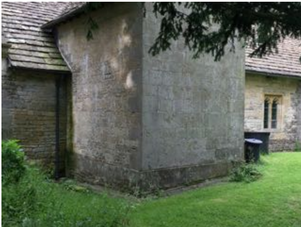
Figure 25 & 26 ~ North elevation of Newman chapel above and north east corner below. The perimeter footprint of the chapel is clear however algae on the east wall adjacent to the down pipe implies there might be an issue with the correct functioning of the rainwater goods.
