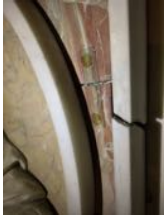
Figure 8 ~ An historic tell-tale across a crack to the upper east of the monument is in tact and appears to still be adhered. This implies that the movement has ceased. However the date of the tell tale is unknown.
