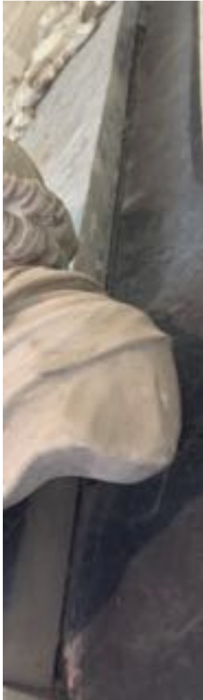
Figure 7 ~ Obelisk back plate detaching along full height on east side.
