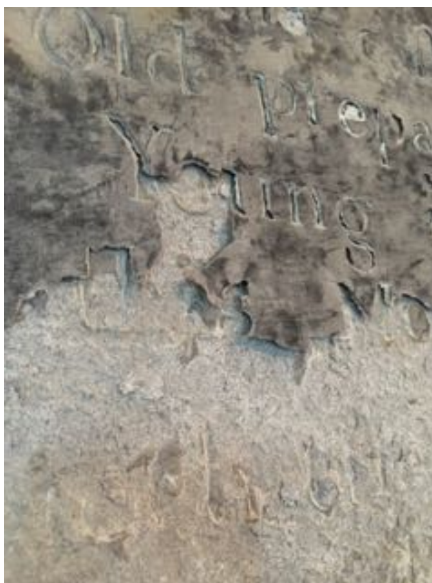
Figure 17 ~ Laminating surface of inscription panel.
