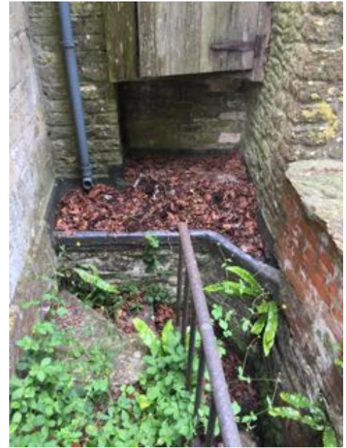
Figure 28 ~ Detail of area to west of Newman Chapel. A build up leaves at base of down pipe.
