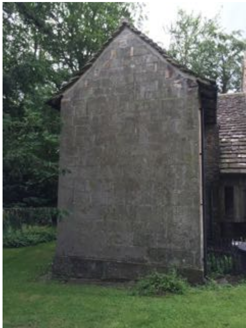
Figure 25 & 26 ~ North elevation of Newman chapel above and north east corner below. The perimeter footprint of the chapel is clear however algae on the east wall adjacent to the down pipe implies there might be an issue with the correct functioning of the rainwater goods.
